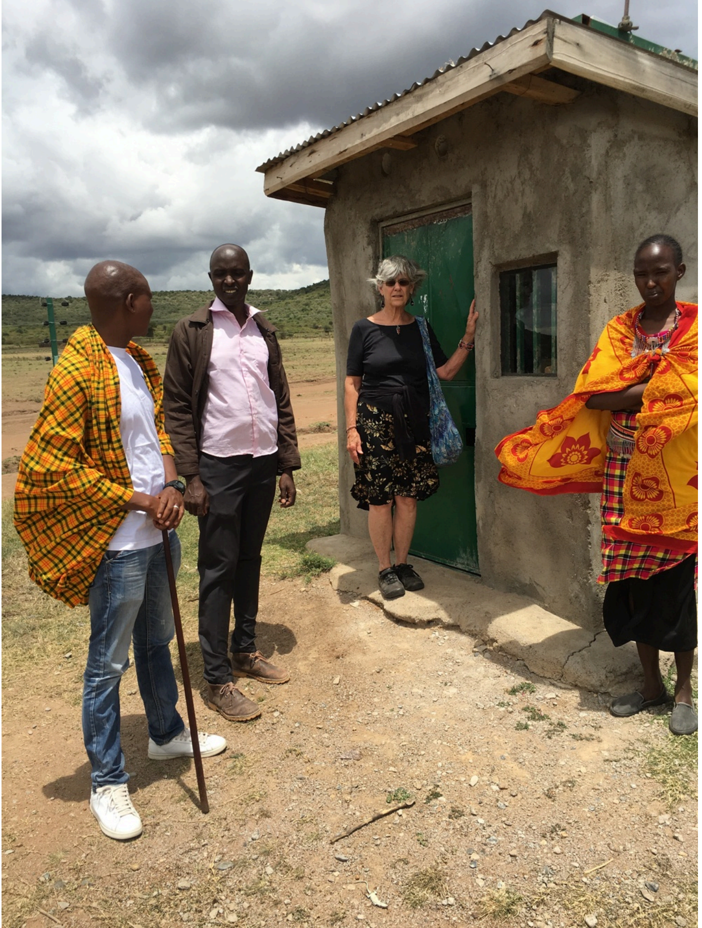
power house for electric fence
